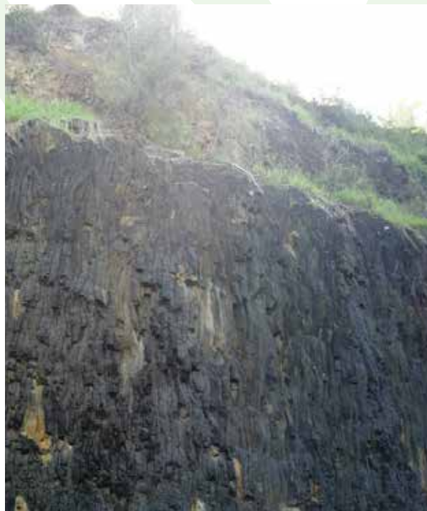
Example of steep terrain along the cliff side of the LFA infested area
